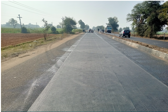
Laying of MacGrid AR
