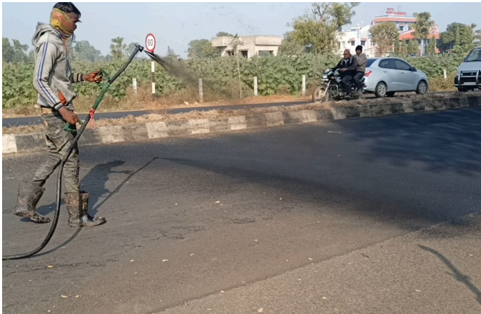
Application of Tack Coat
