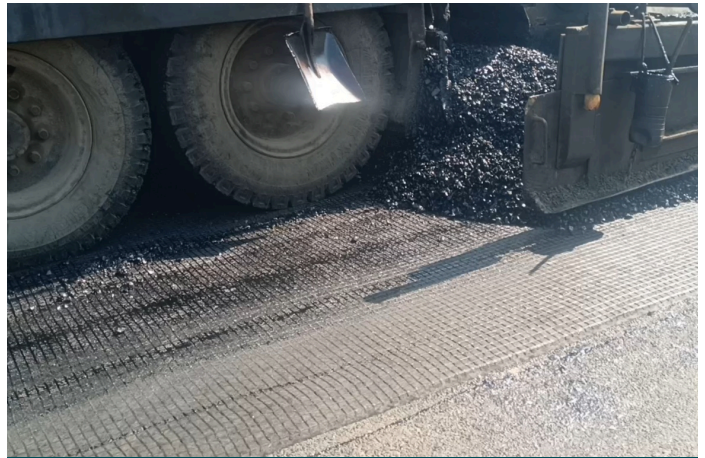
Laying of overlay
