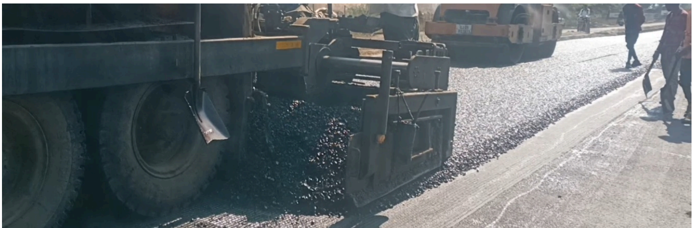
Compaction of Overlay
