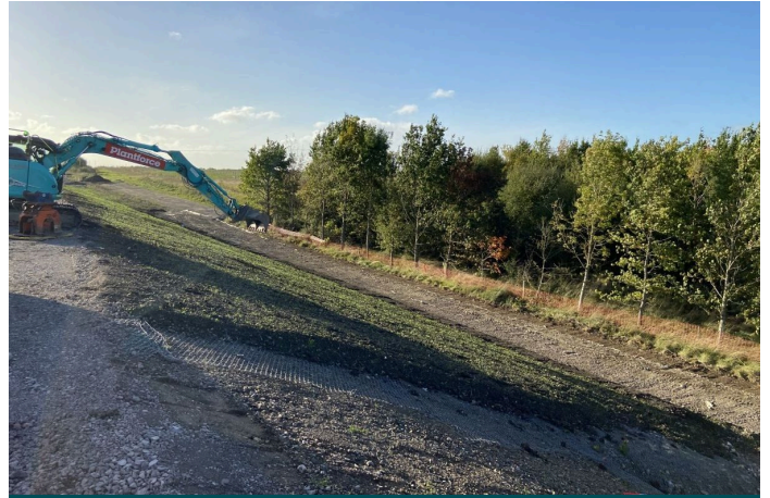
Area covered with the protective mesh
