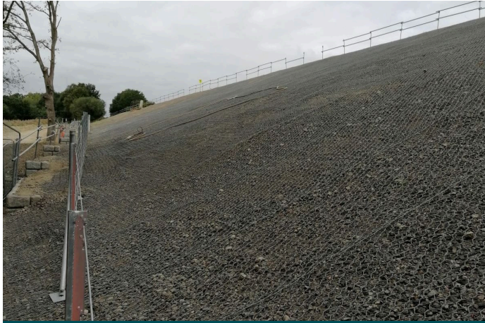
Anti-burrowing DT Mesh deployed and secured
