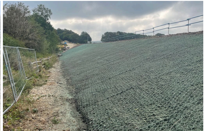
Anti-burrowing DT Mesh spread across rail embankment
