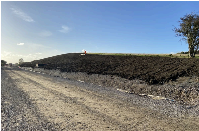
RAILWAY EMBANKMENT BURROWING PREVENTION
