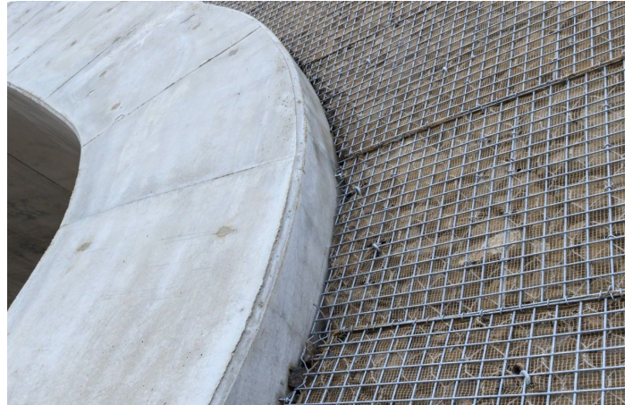
Construction phase: shape detail
