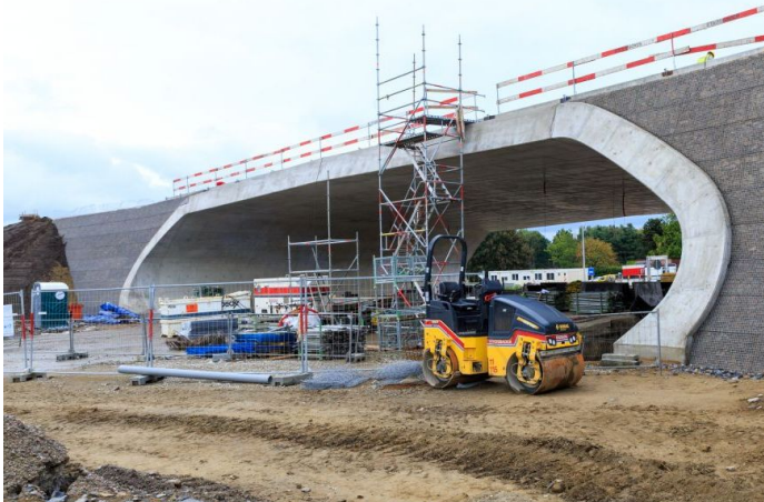
End of the construction: front view
