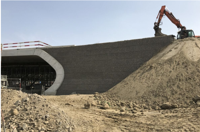
Construction phase: front view
