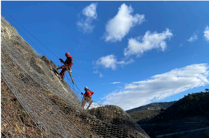
During the construction
