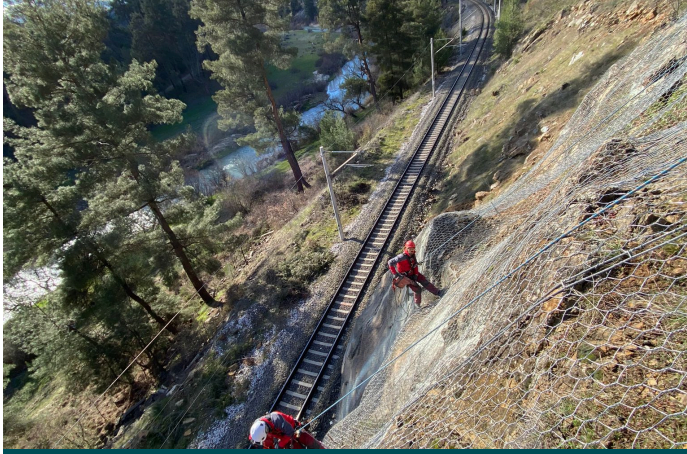
During the construction
