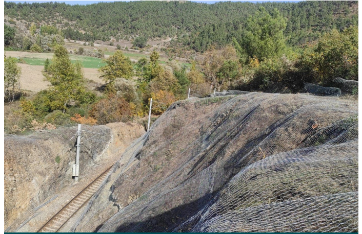
After the installation of HEA Panels
