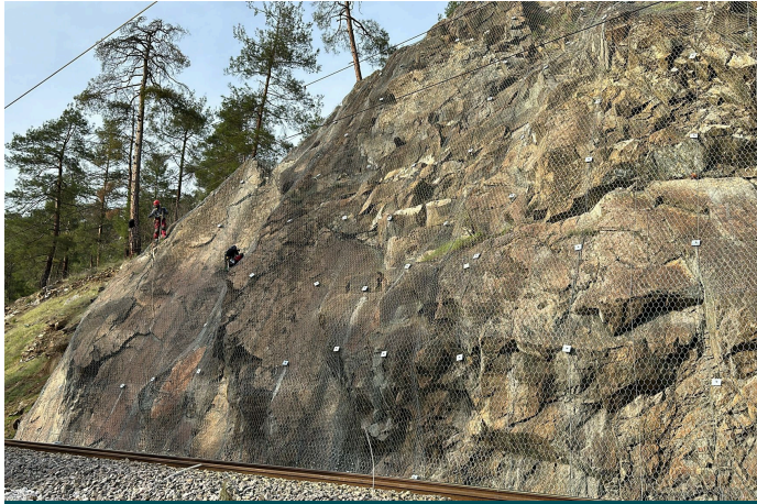
After the installation of HEA Panels
