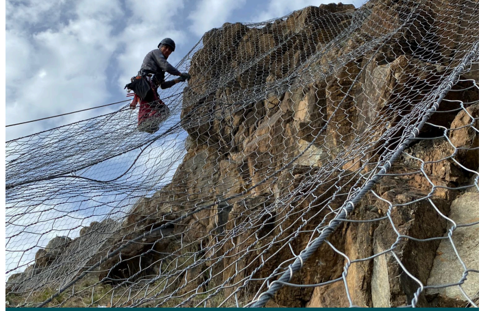
During the construction
