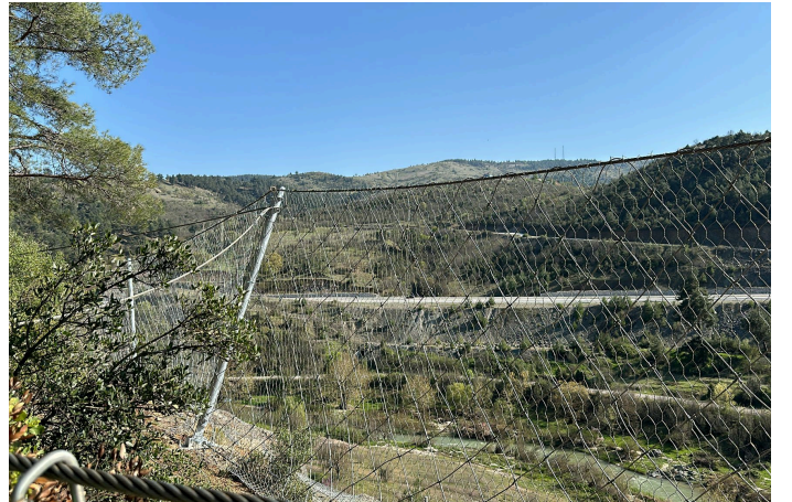
After the installation of dynamic barrier RB 750
