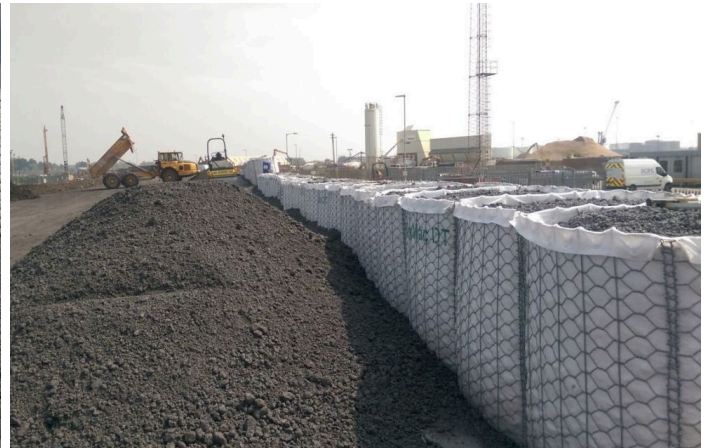
Backfill placement behind the structure
