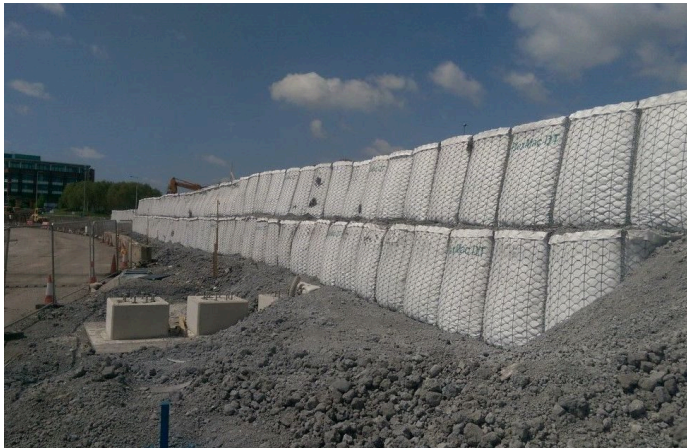
FlexMac DT temporary structure
