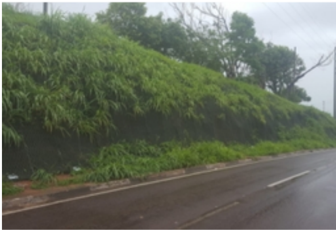
EROSION CONTROL AT LEUWIKERIS DAM - PACKAGE 1_4
