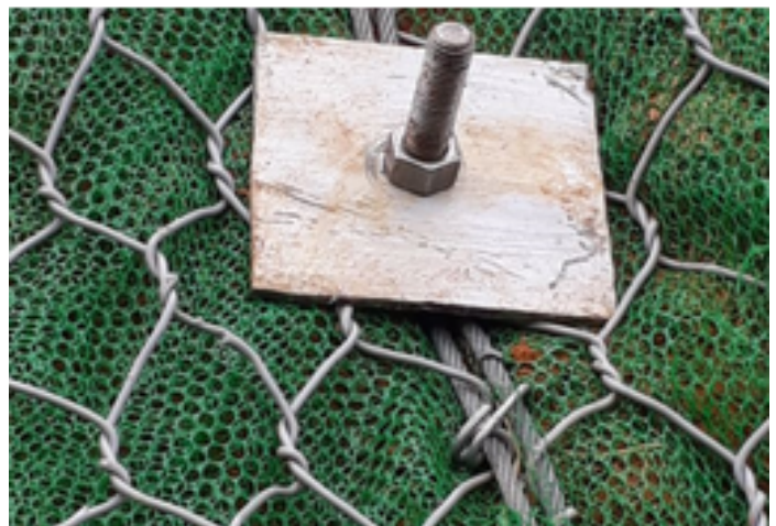
EROSION CONTROL AT LEUWIKERIS DAM - PACKAGE 1_3
