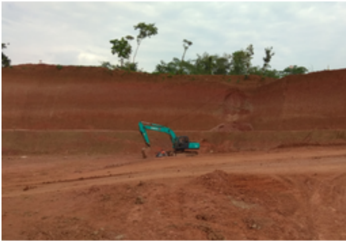
EROSION CONTROL AT LEUWIKERIS DAM - PACKAGE 1_0
