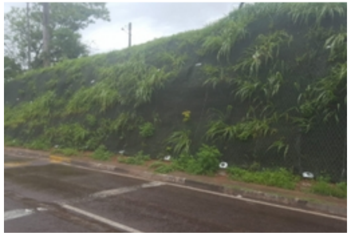
EROSION CONTROL AT LEUWIKERIS DAM - PACKAGE 1_5
