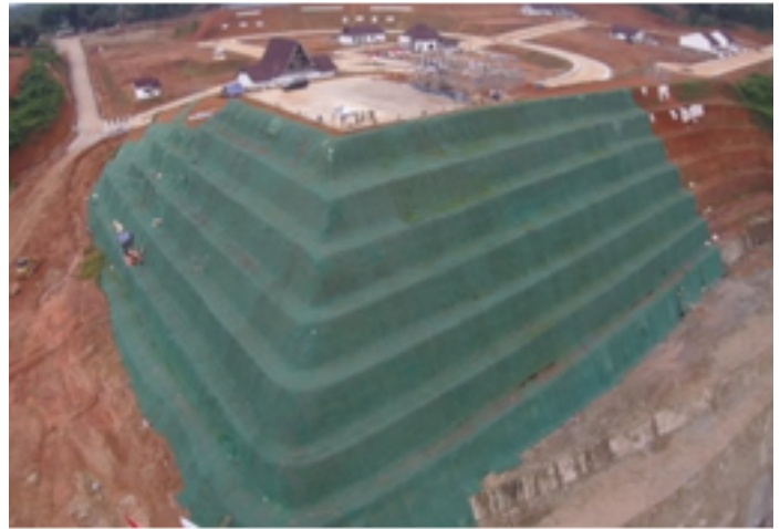
EROSION CONTROL AT LEUWIKERIS DAM - PACKAGE 1_1
