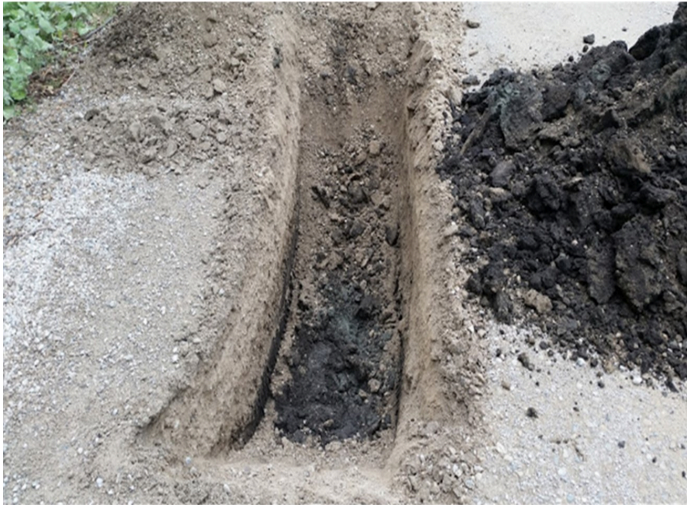
Detail of the black native soil at the base of the road
