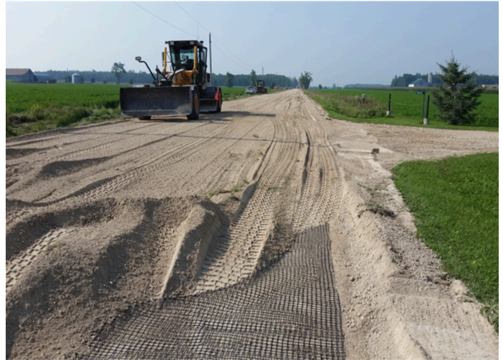
Detail of granular A on top of MacGrid EG-30S
