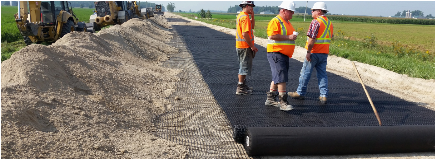
Detail of MacGrid EG-30S and MacTex Mx-225 placing
