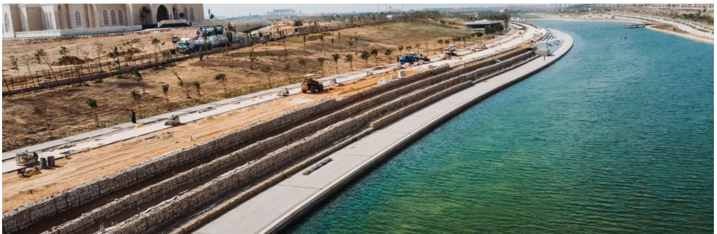
Distant view of Terramesh MSE wall along the banks of Green river
