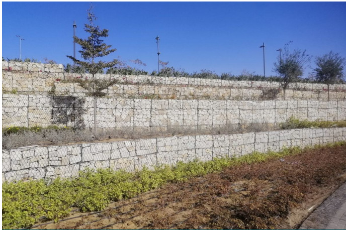
Close view of the Terramesh MSE wall with plantation
