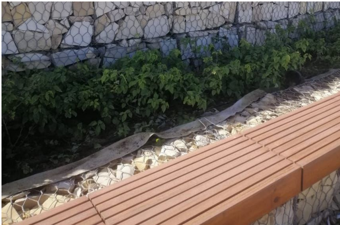
Close view of the Terramesh MSE wall with bench
