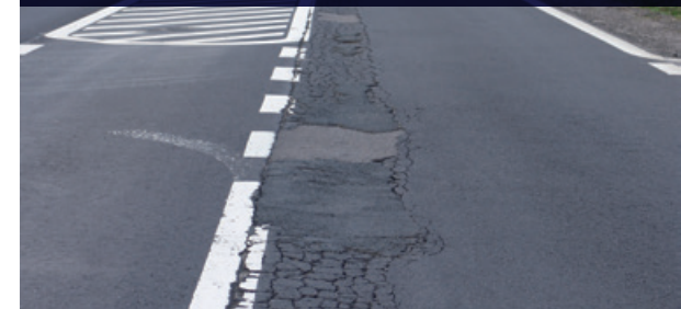
Fatigue cracking
