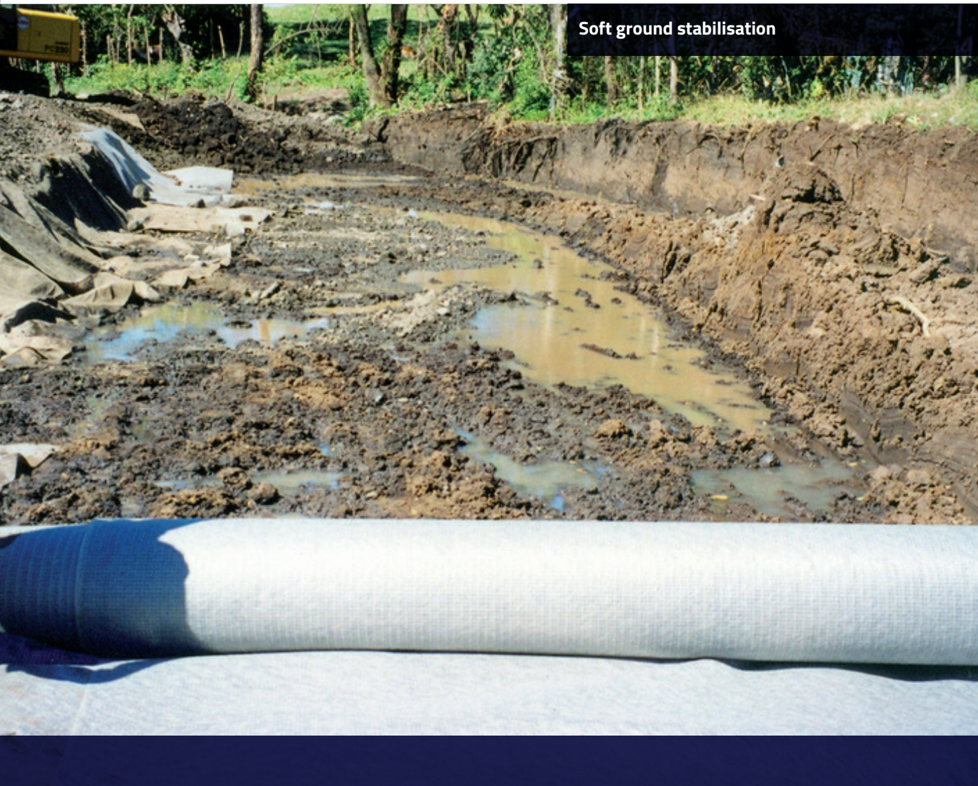
Access over wet/soft ground
