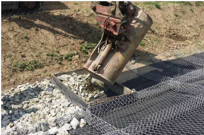
During the installation: stone-filling operation
