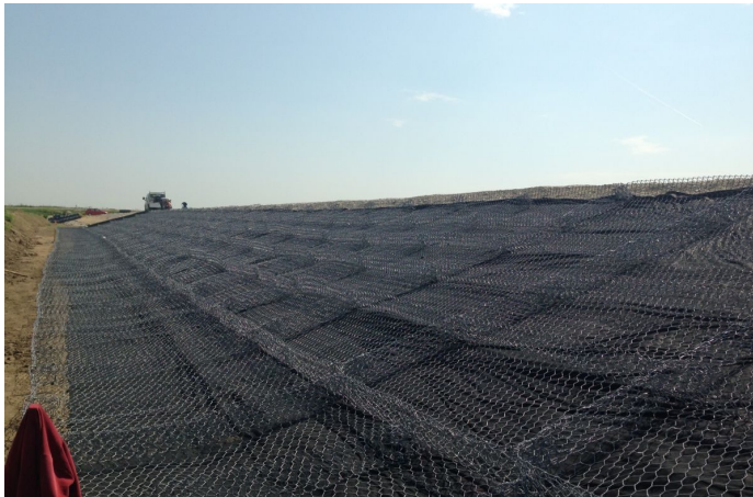
Installation phase: detail of the empty units
