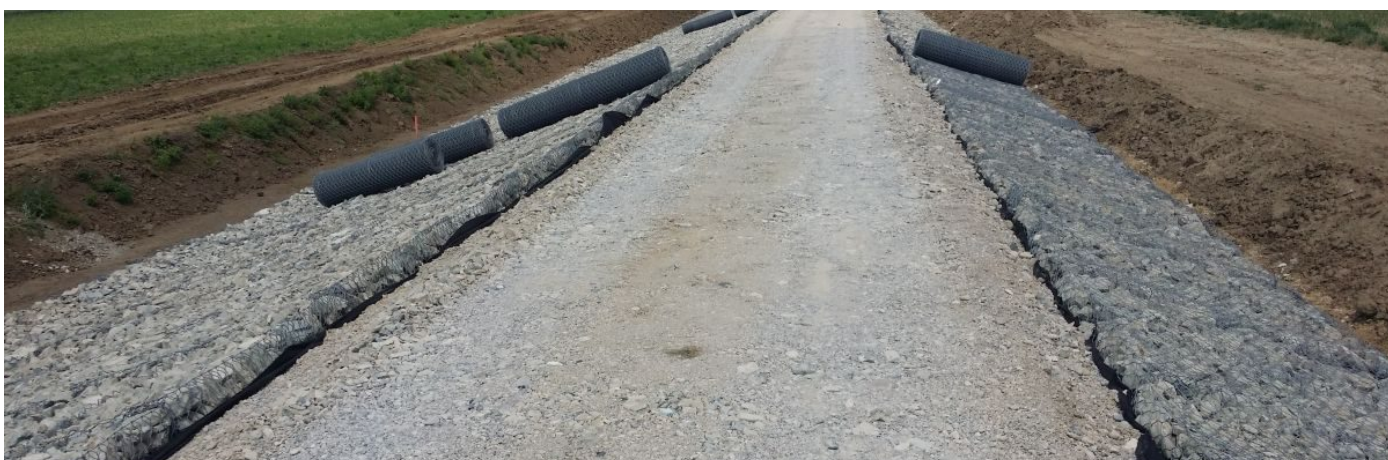
After the installation
