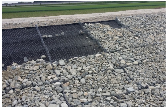
During the installation: stone-filling operation
