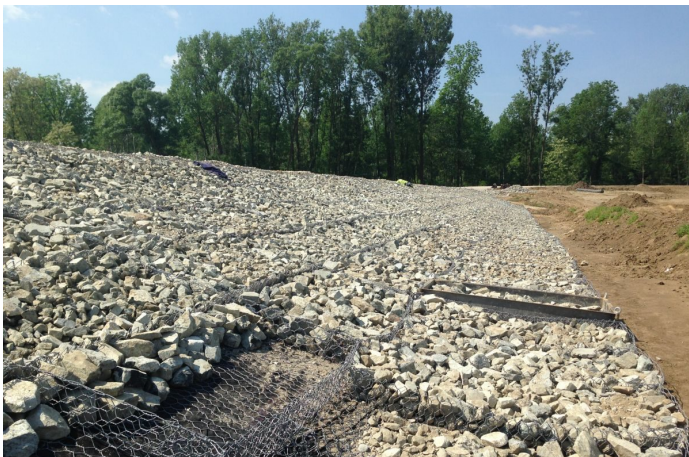
During the installation
