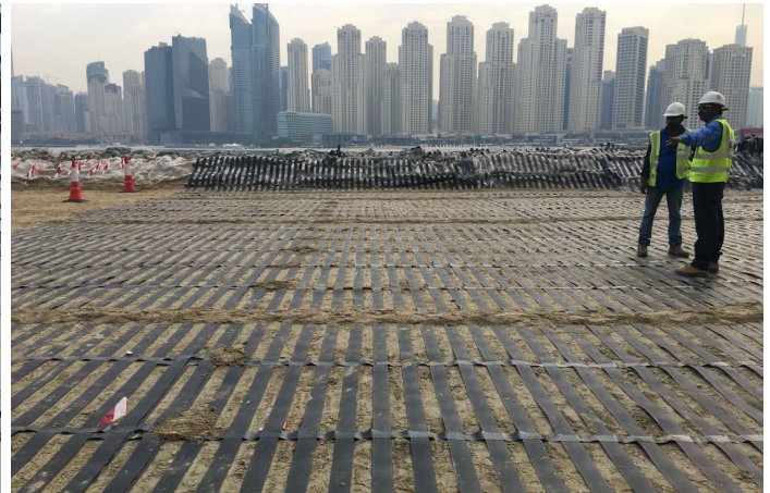
During construction: close view of laid Paralink 300 geogrid
