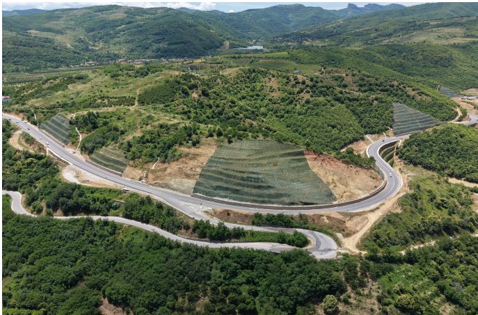
Slope protection &amp; Erosion Control
