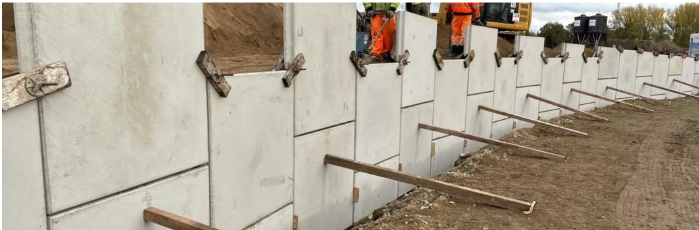
Construction phase: panels installation
