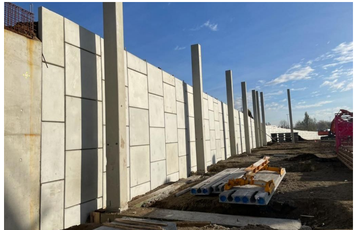
Construction phase: connection between the panels and the
