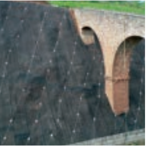
6 Soil Nailing and Surface Protection
