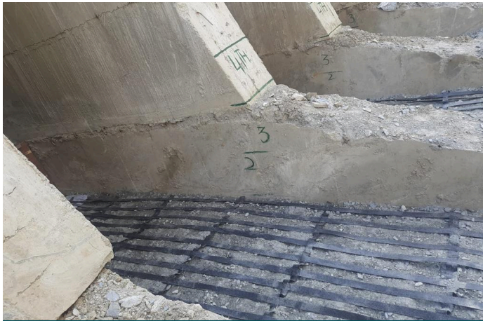
Laying of ParaLink
