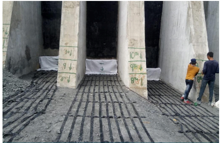
Placing of Geotextile and Laying of ParaLink
