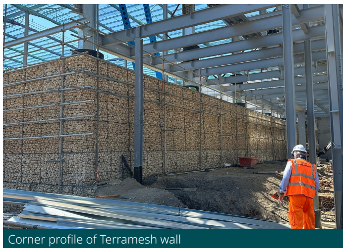
Terramesh wall in the final stages
