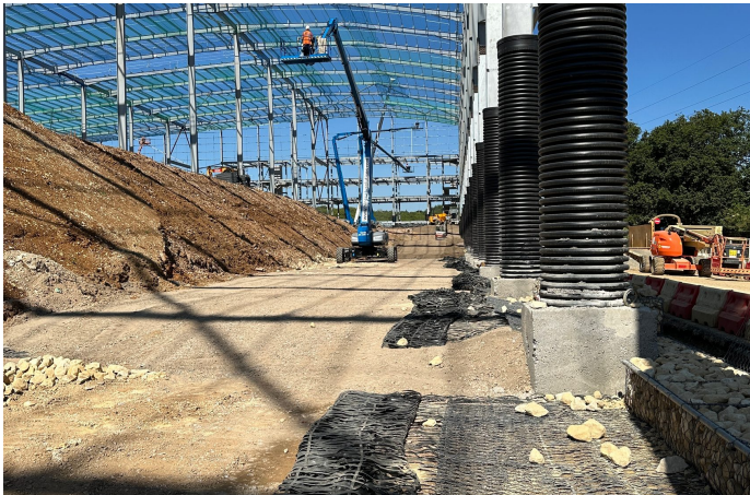
Terramesh units with ParaGrid geogrids reinforcement being
