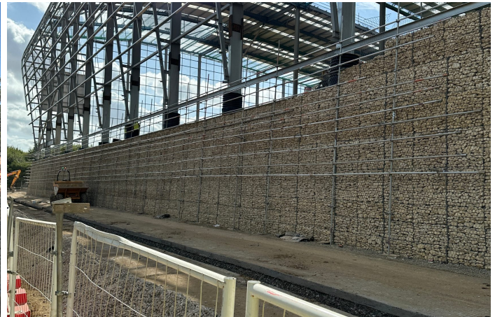
Terramesh mid-construction
