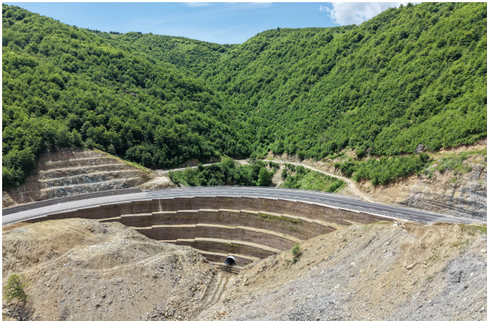
Reinforced soil wall back to back Hmax=41m
