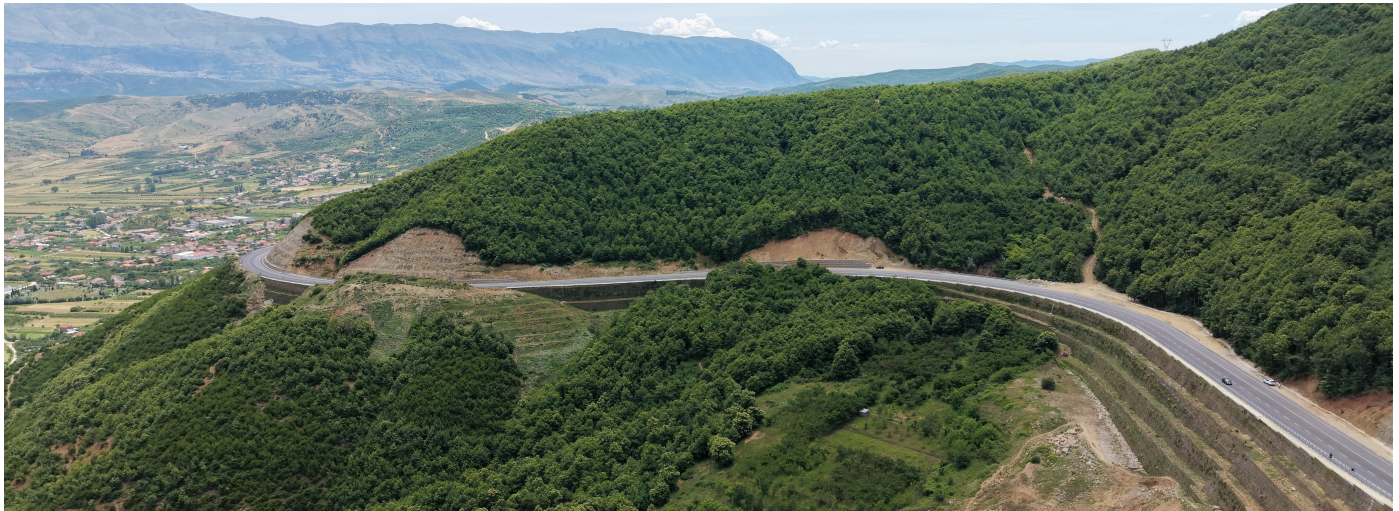
Reinforced soil walls
