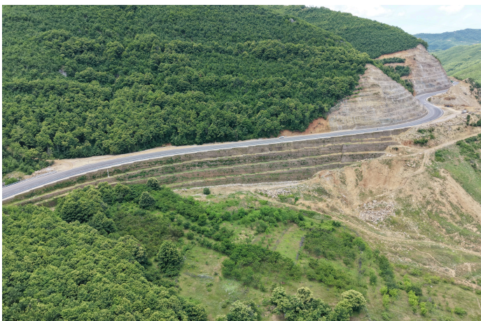
Reinforced soil wall Hmax=30m, L=380m
