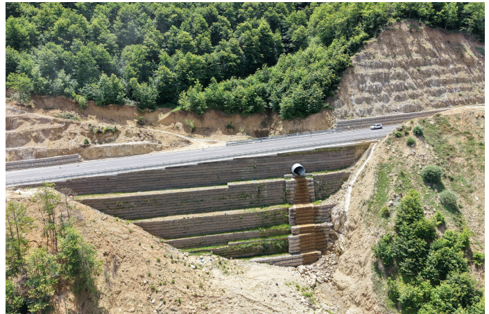
Reinforced soil wall back to back Hmax=31m
