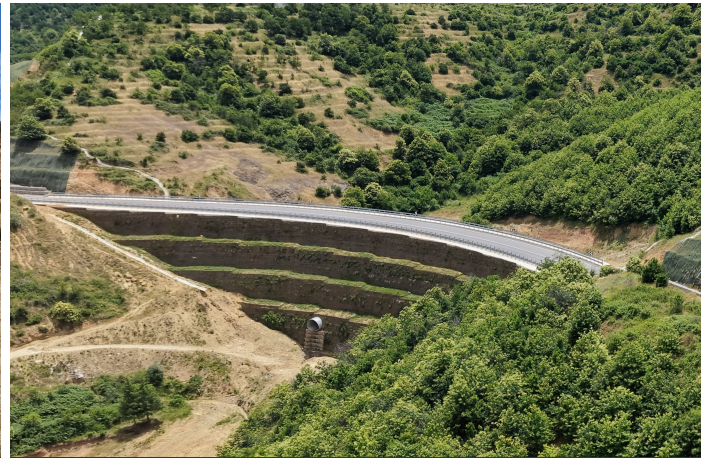
Reinforced soil wall back to back Hmax=30m
