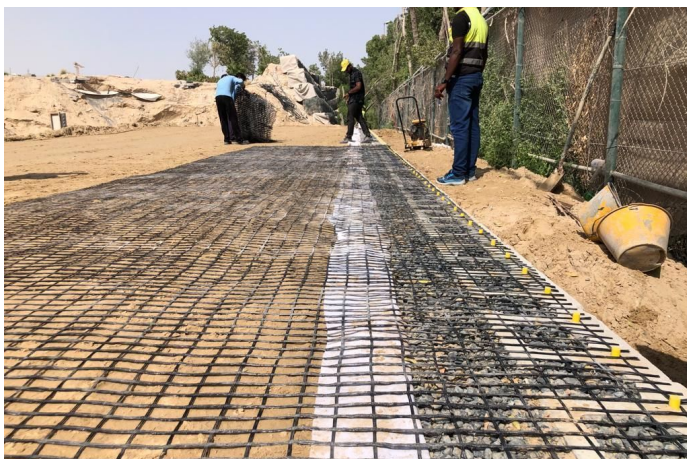
MacWall installation in progress
