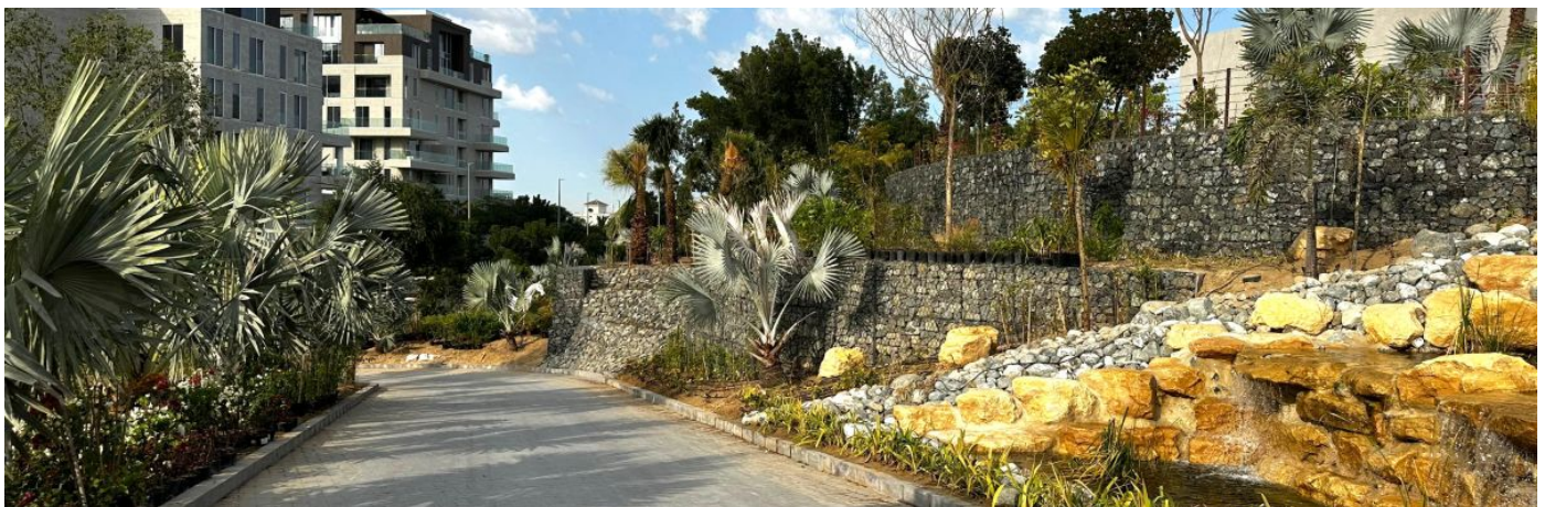
Completed Terramesh MSE wall with plantation works
