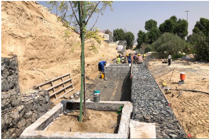
Terramesh MSE wall in progress
