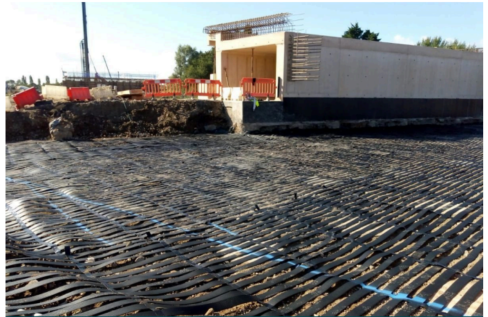
Cranes and piling rigs over the MacTex W1 reinforced
