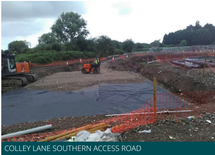
MacTex W1 S laid over soft clay sub-strata
