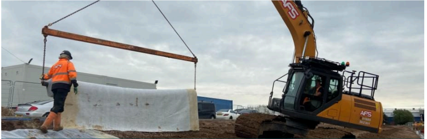
Macline GCL placed in drain trench to seal under filter drain.
