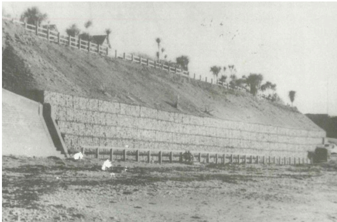
After construction in 1971
