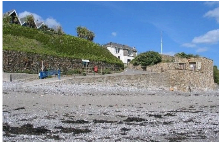
View of the sea defence wall as it now appears
