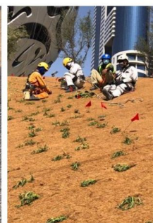
Biomac Installation & Plantation Works
