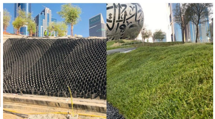
During construction: Macweb geocell (before & after)
