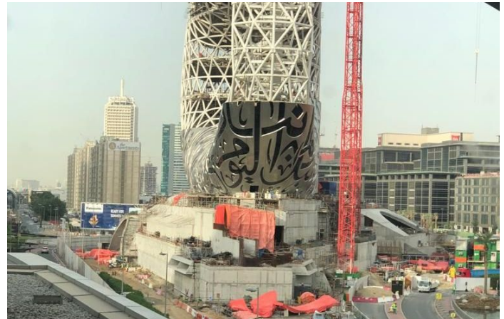
During construction: embedded building before covering
