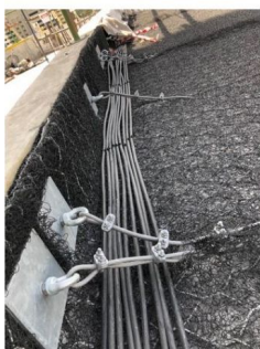
Macmat HS & Concrete Anchor Installation
