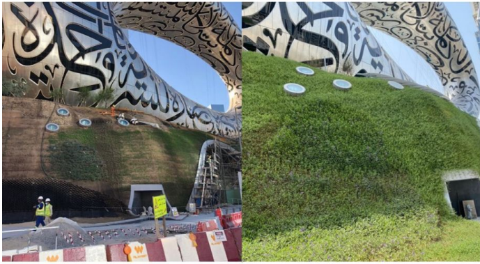
During construction: Green Terramesh soil slope (before &
