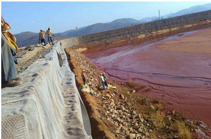
PHOTOGRAPH SHOWING GCL INSTALLATION OVER THE
