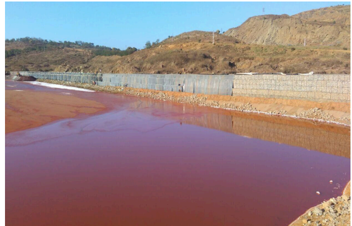
CONSTRUCTION OF GABION WALL ALONG WITH
