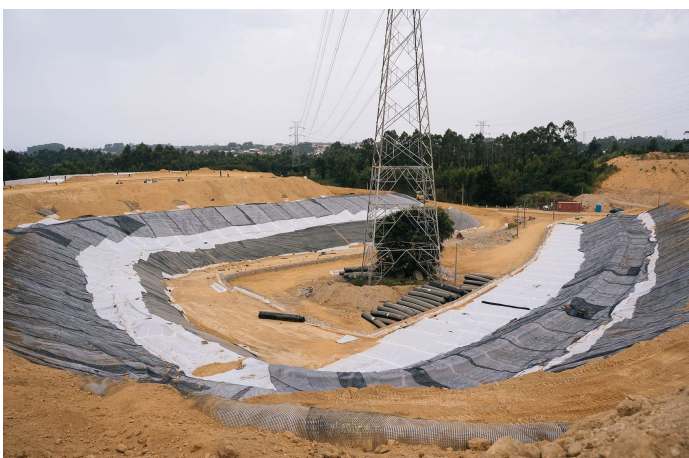
Installation of MacDrain W and MacGrid WG
