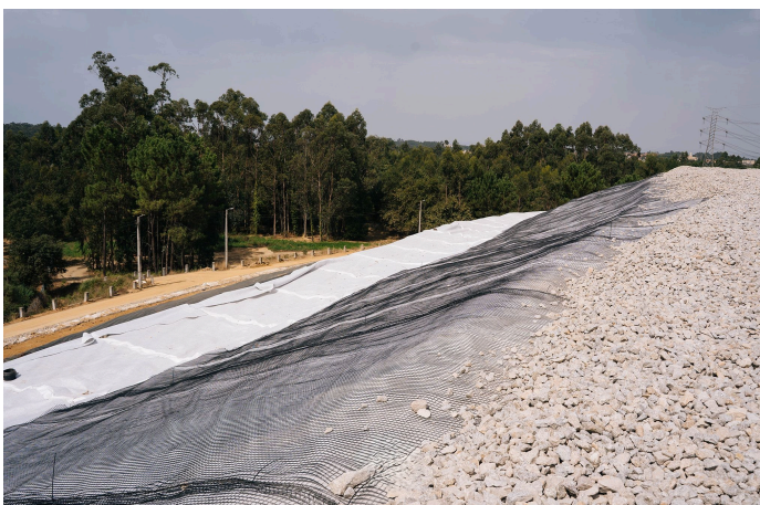
Installation of MacGrid WG geogrid
