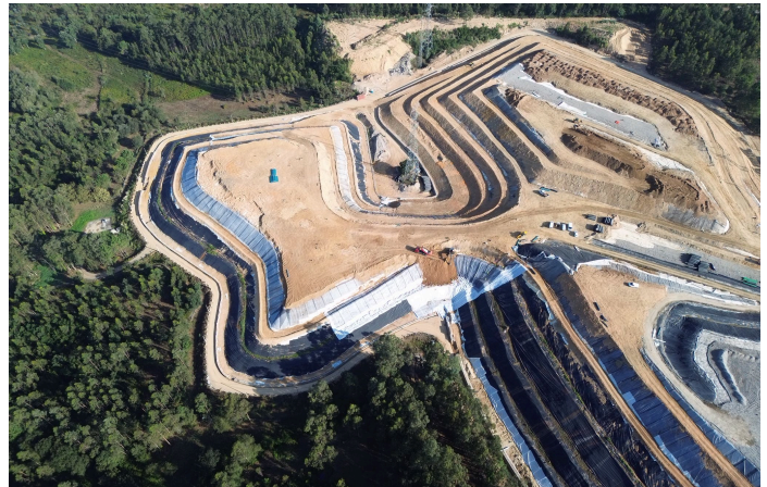
Aerial view of the landfill site looking west-east
