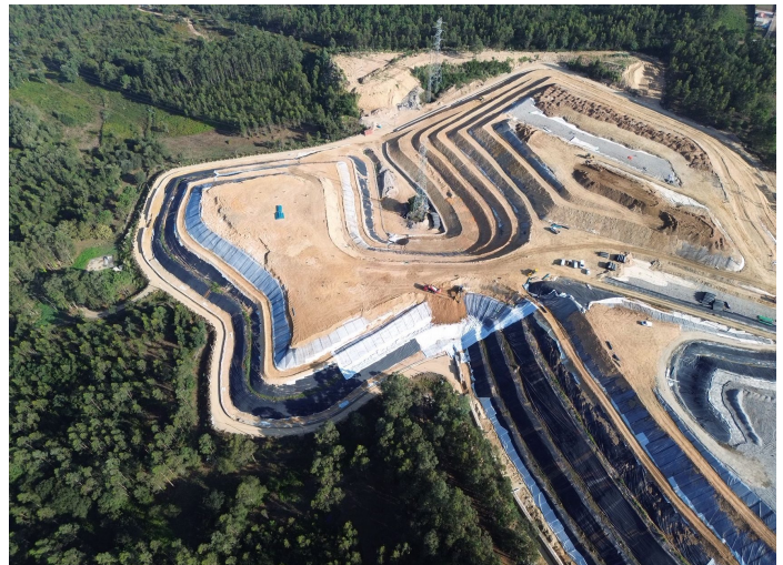
Aerial view of the landfill site looking west-east
