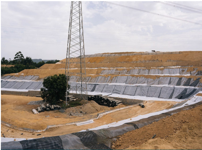
View of the slopes and embankments of the landfill site
