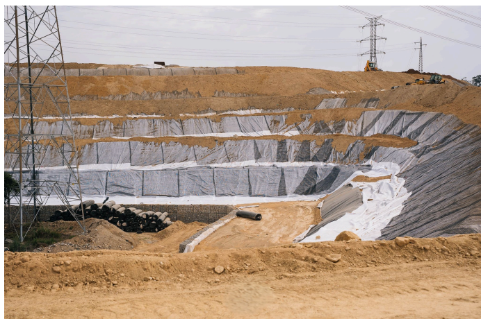
Gabion wall at the foot and slopes of the landfill
