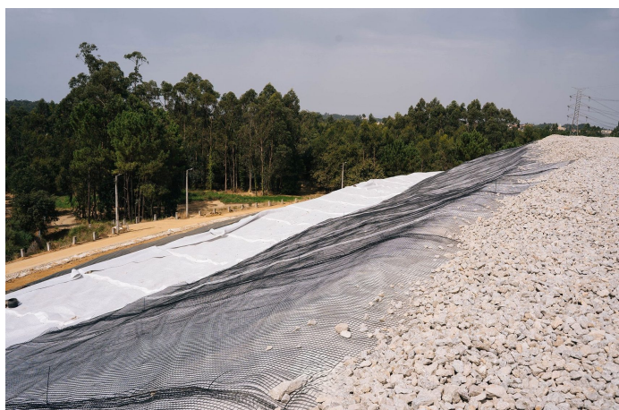
Installation of MacGrid WG geogrid
