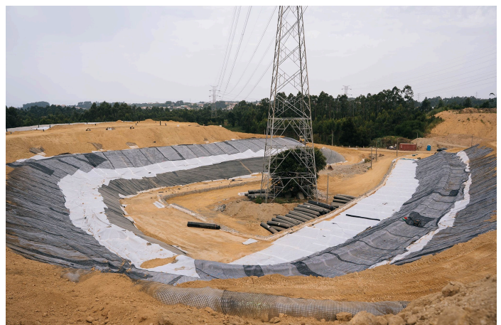
Installation of MacDrain W and MacGrid WG
