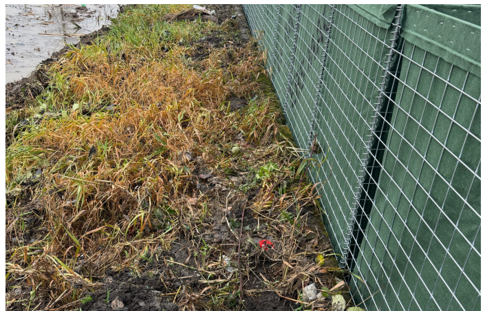
After: White River Flood Protection Barriers
