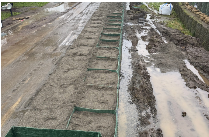
During: Emergency Breach Repair Protecting Pacific Park
