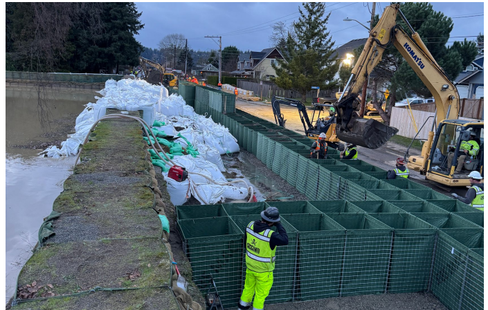
During: Emergency Breach Repair
