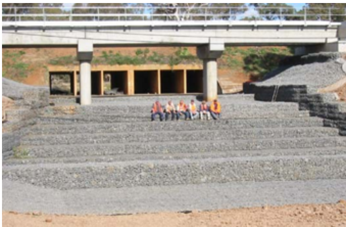
End Perspective of Drop Structure
