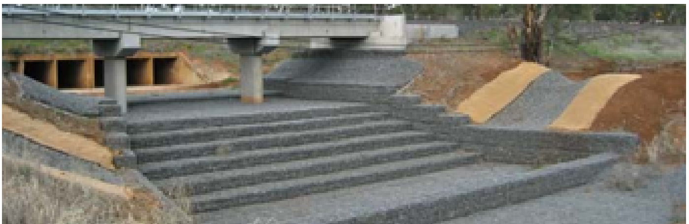
Completed Drop Structure
