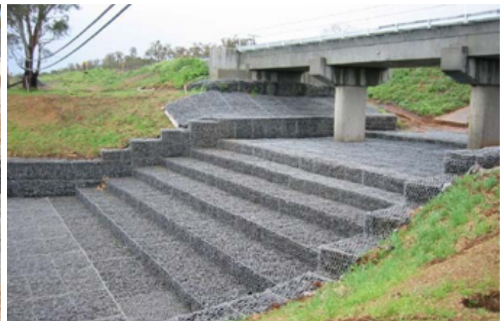
Completed Drop Structure
