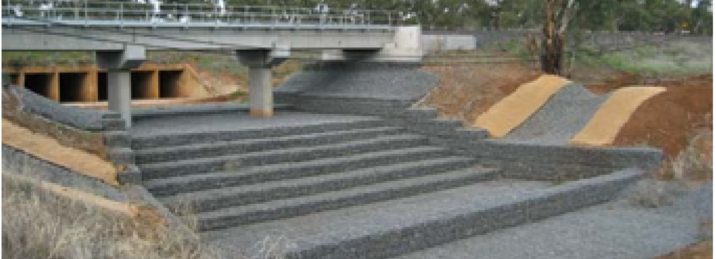
Completed Drop Structure
