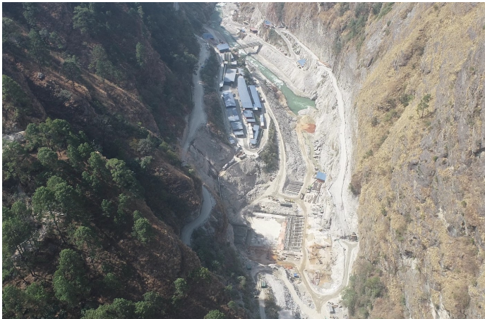
Fig-1 Initial site condition-Top view
