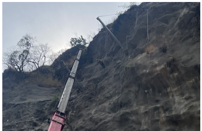
Fig-4 Rockfall Barrier installation
