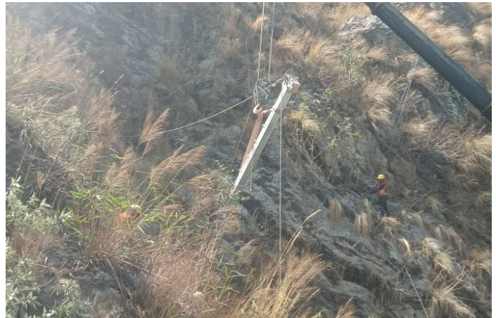
Fig-2 Rockfall Barrier installation
