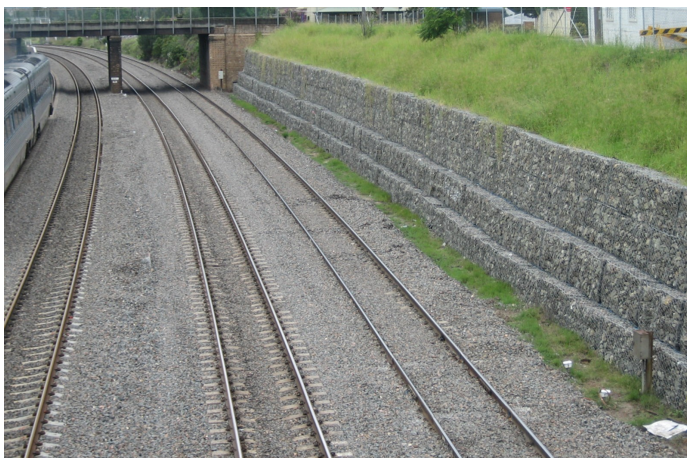
After construction - Mar 2007
