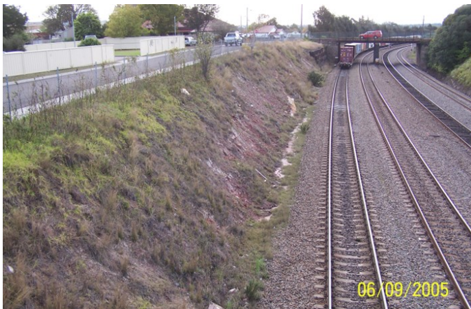
Before construction - Sep 2005
