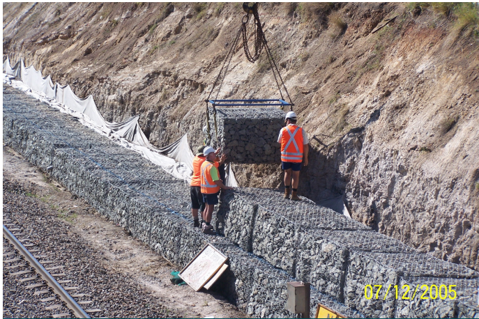
During construction - Dec 2005
