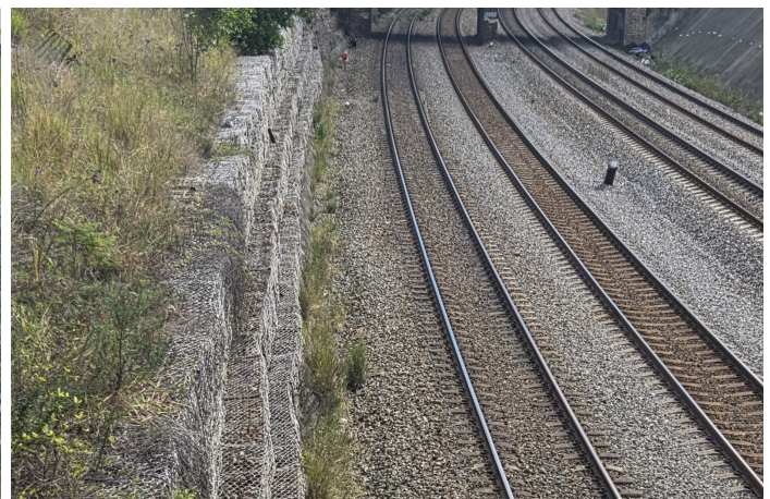
After construction - Mar 2026
