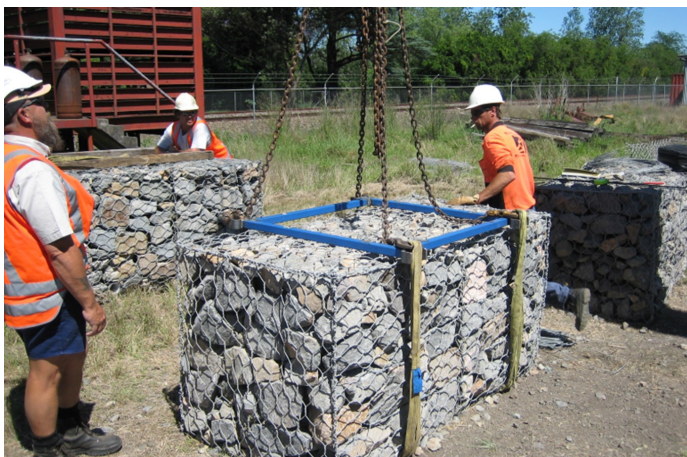
Lifting procedure with slings and frame - Nov 2005
