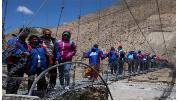
Hanging Bridge : Hilsa
