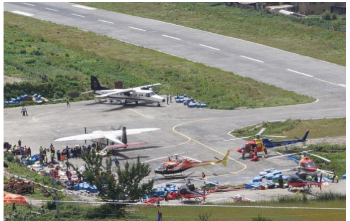
Simikot Runway & Helipad
