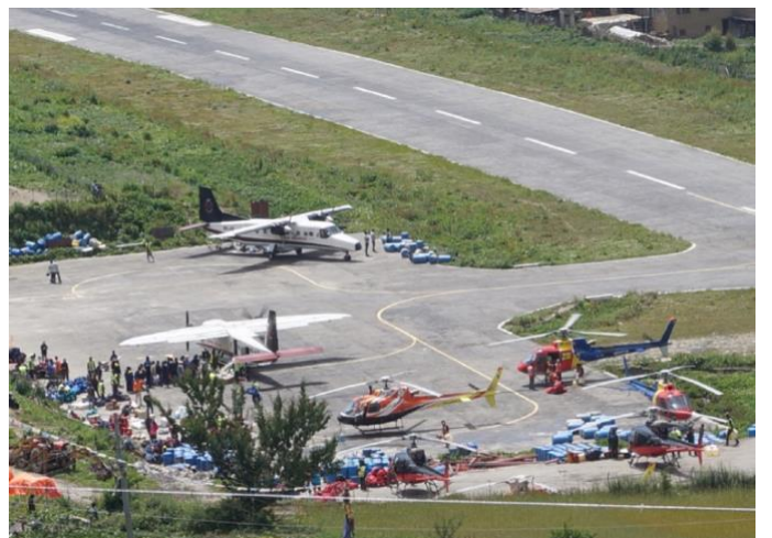
Simikot Runway & Helipad
