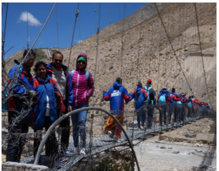
Hanging Bridge : Hilsa
