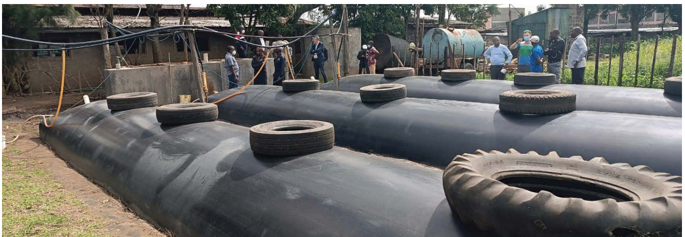
Community-Based Biogas Facility During On-Site Technical Inspection and Evaluation
