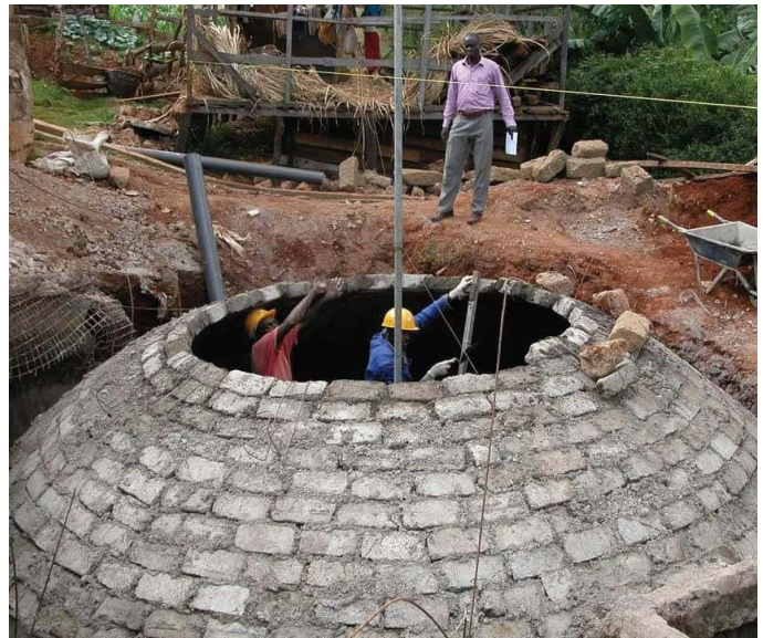
A fixed dome biodigester under construction
