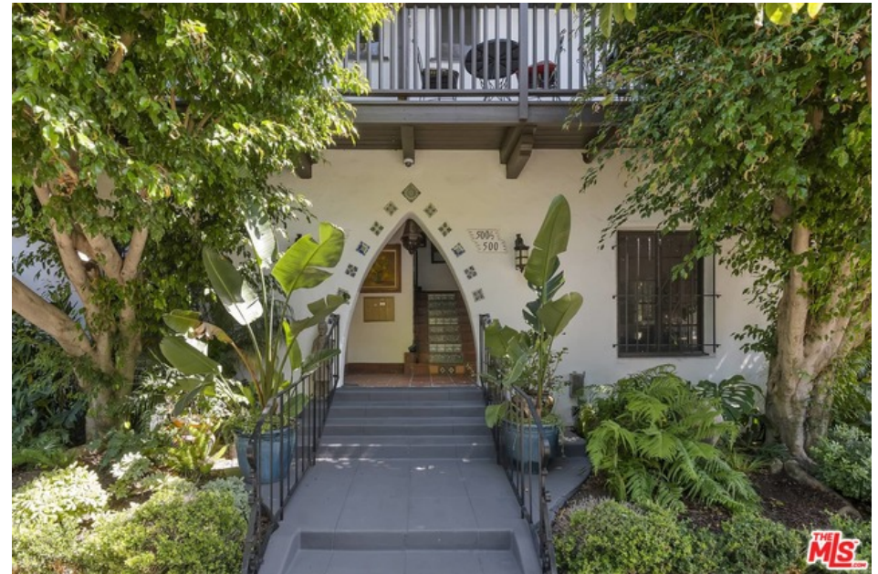
The entrance to an older building that has been converted to a TIC, and which includes units listed by Stanley. Credit: Christopher Stanley and Vanguard Properties
